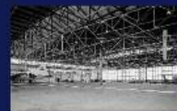
Interior of building 4 (P-13)
