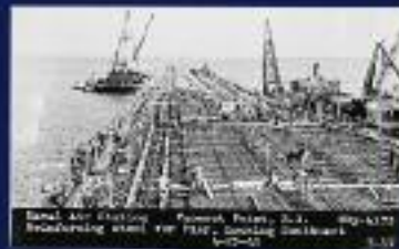
Reinforcing the pier
